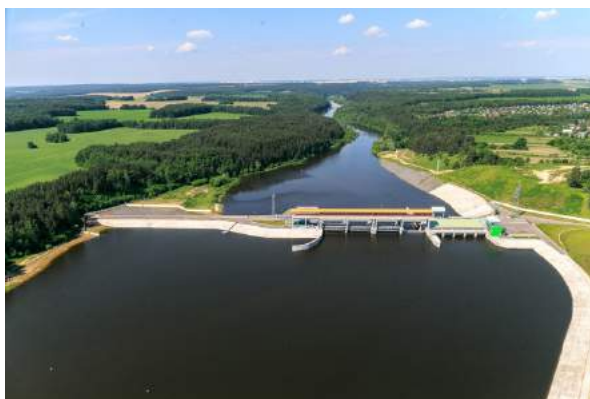
Figure 1. Grodno hydroelectric power station
