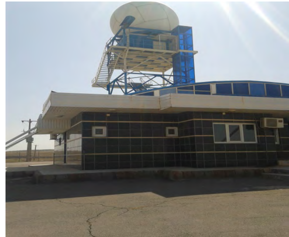
Figure 1. The Sahand radar
